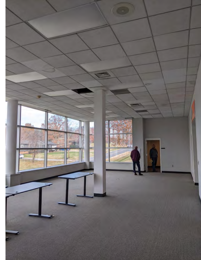
Upper level – secondary open office area
