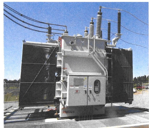
Figure 6. GSU Transformer with Secondary Containment to Capture any Leaked Oil
