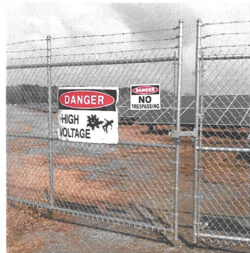
Figure 1. Perimeter Fence with Warning Signs
