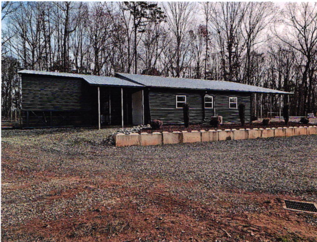
This is from the left side looking at the back left corner of the shop.
